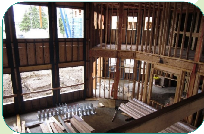
Construction at Rosslyn Terrace
