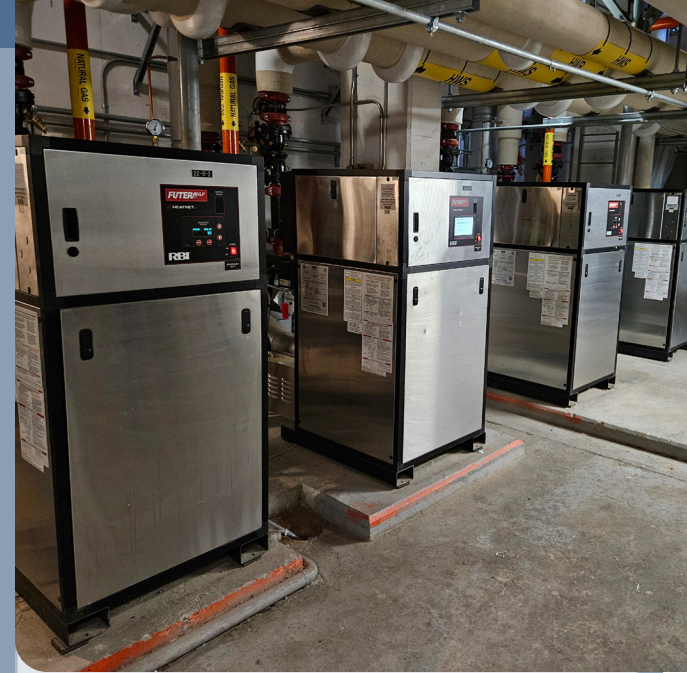
Capital project improvements included boiler replacements for Kiwanis Place .
